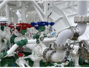
• Manifold onboard "EXCOOL" Transferring the liquefied CO<sub>2</sub> by connecting the loading arm and ship.
